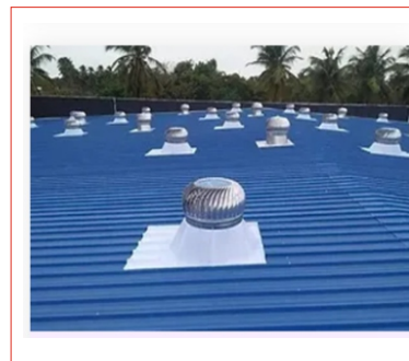
Wind Roof Ventilator
